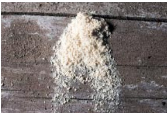
Fig. 4c. Anobiid frass expelled from hole.
