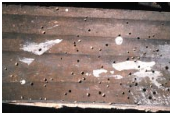
Fig. 4b. Anobiid or deathwatch beetle exit holes.
